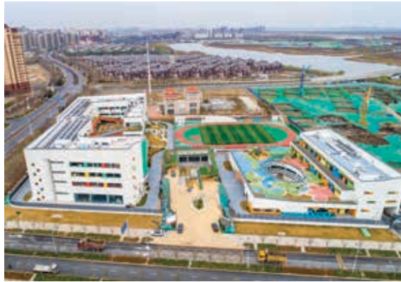
Figure 12-3: Huaxia Future Primary School of Tianjin Eco-City
