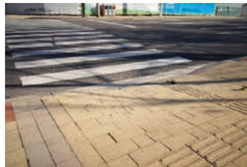
Figure 10-10: Accessibility Design for Crossing Facilities
