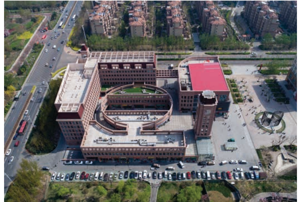
Figure 12-11: Second Community Centre of China-Singapore Tianjin Eco-City
