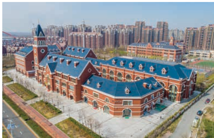
Figure 12-10: First Community Centre of China-Singapore Tianjin Eco-City
