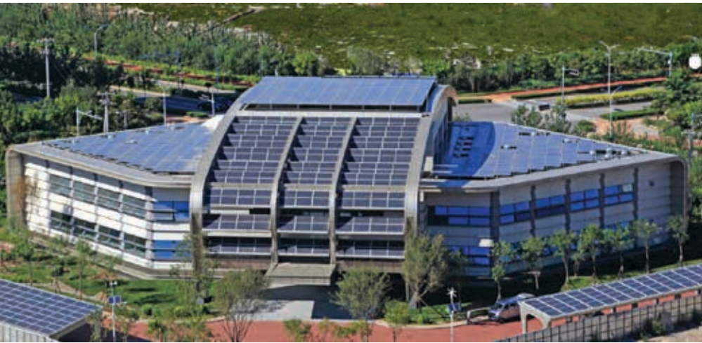
Figure 11-12: TEC Public House Exhibition Centre
