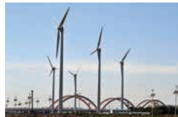
Jiyun River Mouth Wind Power Generation
