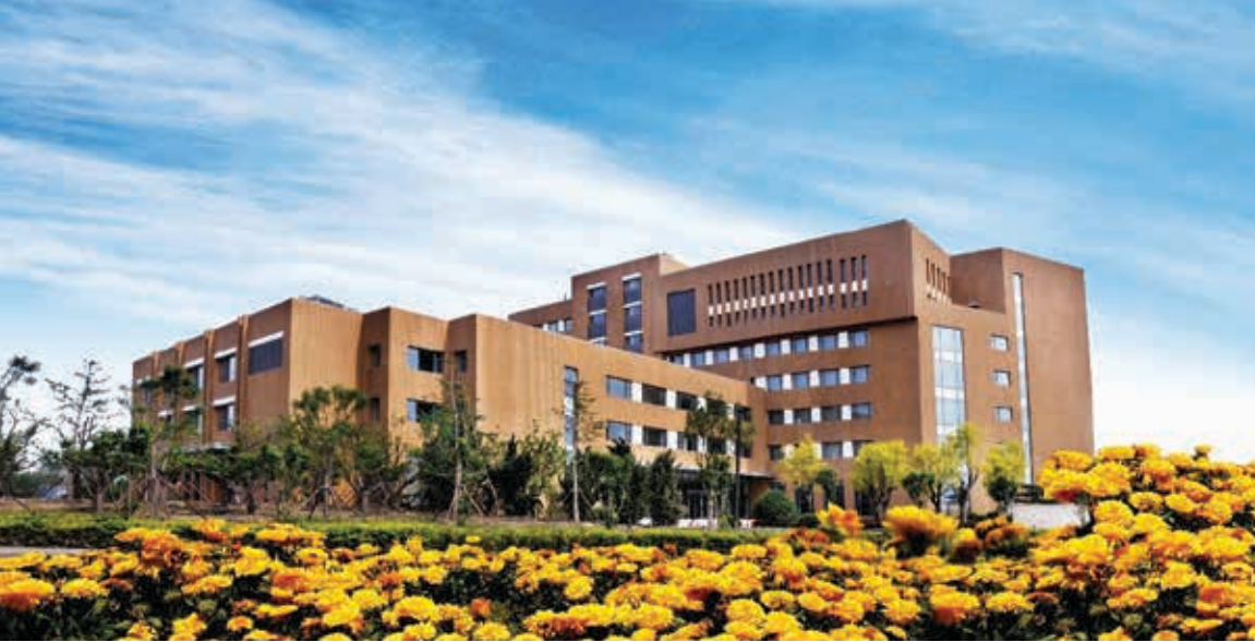
Figure 15-1: Public Utility Operation and Maintenance Centre (Figure 15-1)
