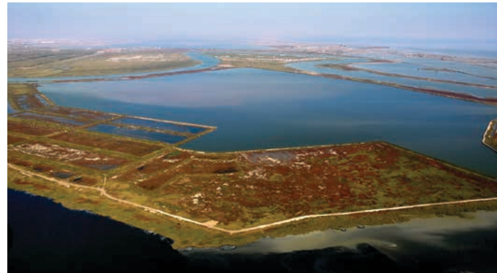
Figure 8-1: Original Appearance of Sewage Reservoir in TEC
