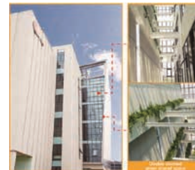
Figure 11-6: Double Skin Structure of Building
