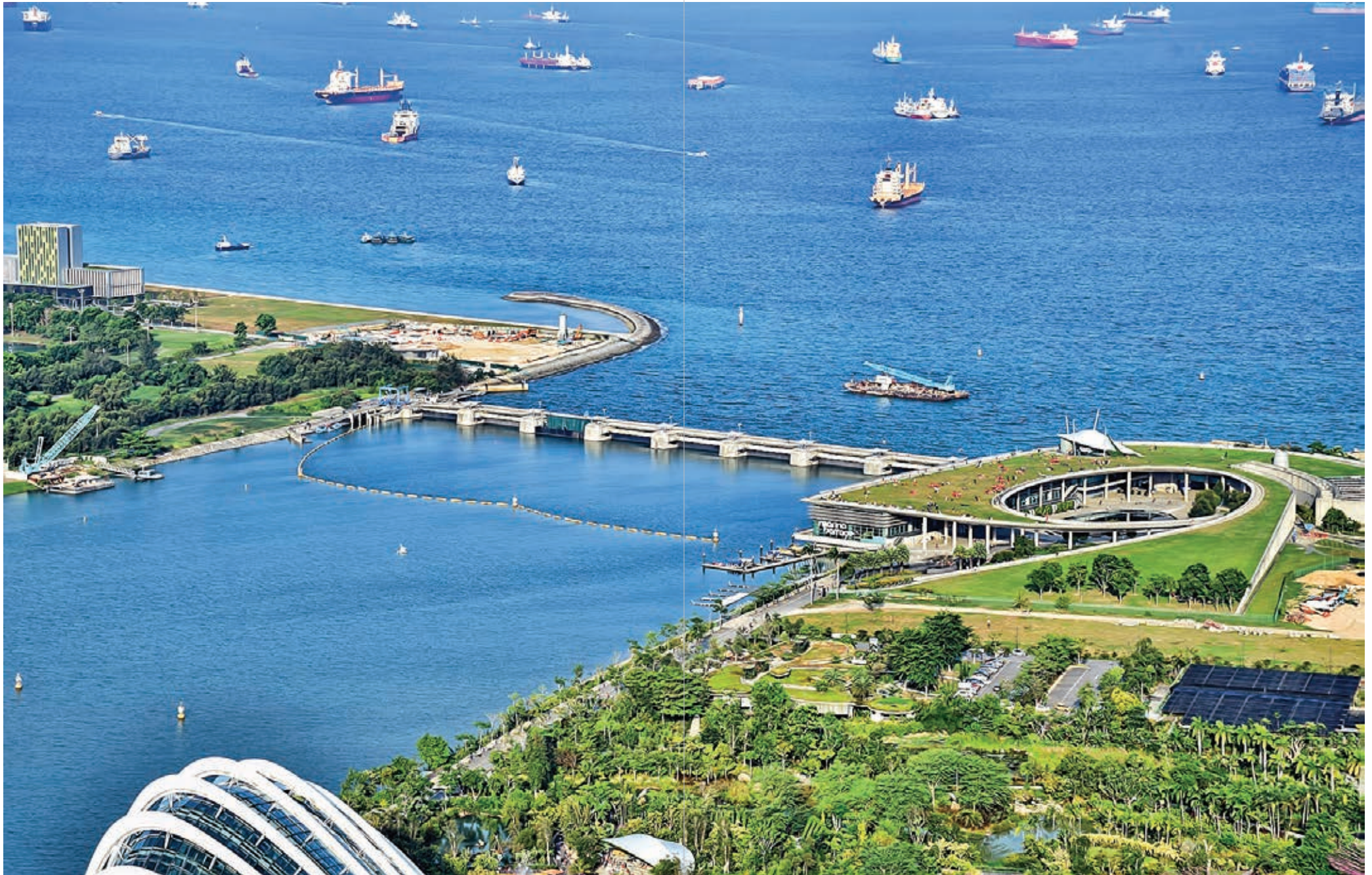
Marina Barrage, completed in 2008, created Singapore's 15th reservoir with a catchment of 10,000 ha, and is part of the flood control measures for low lying areas in the Central Business District.
