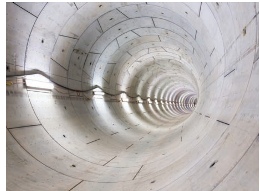
Stamford Diversion Canal (bottom) and the inside of the Stamford Detention Tank (top).
