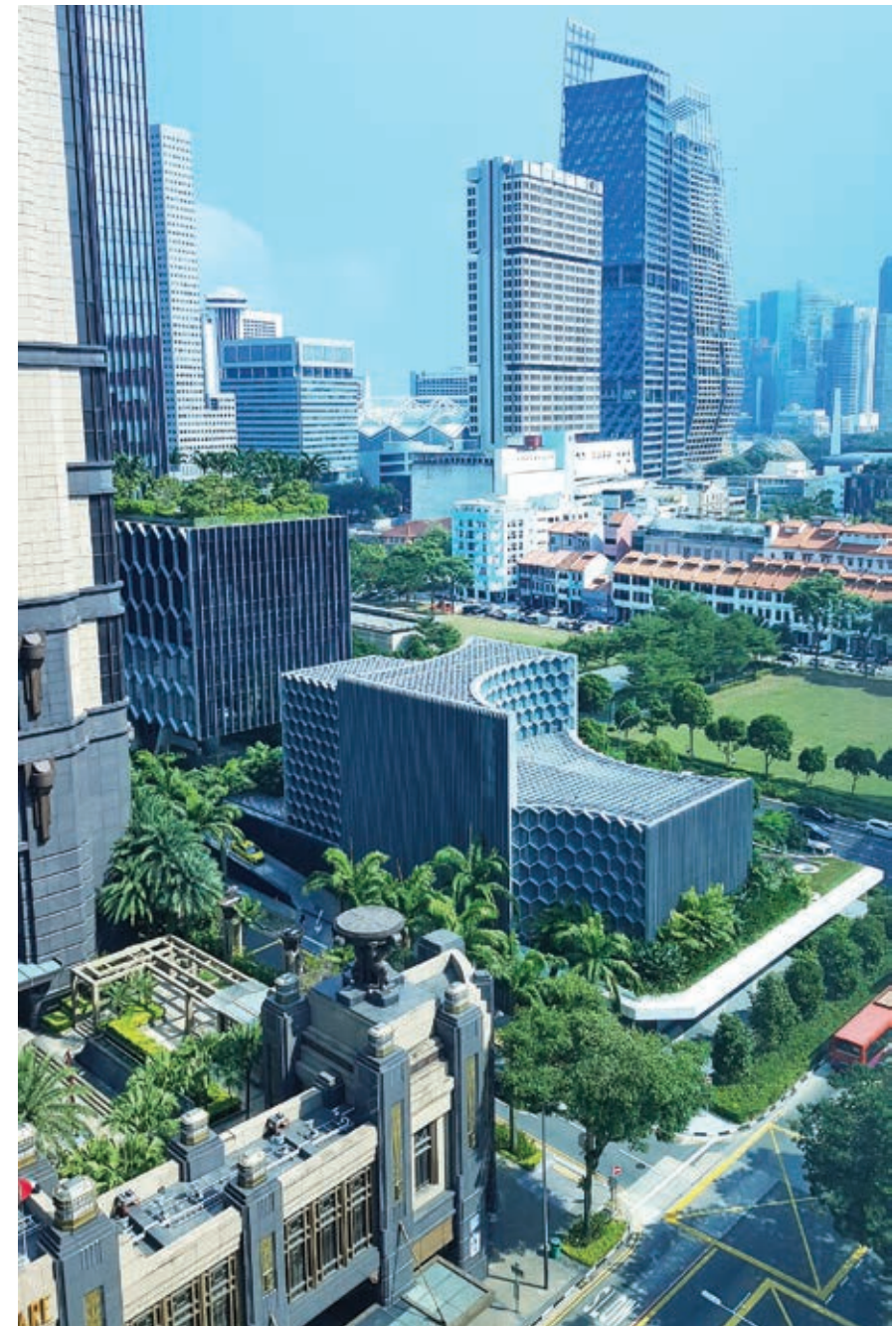
Vertical greenery is increasingly used to manage and delay stormwater runoff and address urban heat island effect in Singapore.
