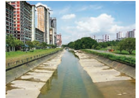
Before, Bishan and Ang Mo Kio neighbourhoods were divided by this concrete canal. The waterway was re-naturalised and integrated with the adjacent park, using ABC Waters design features.
