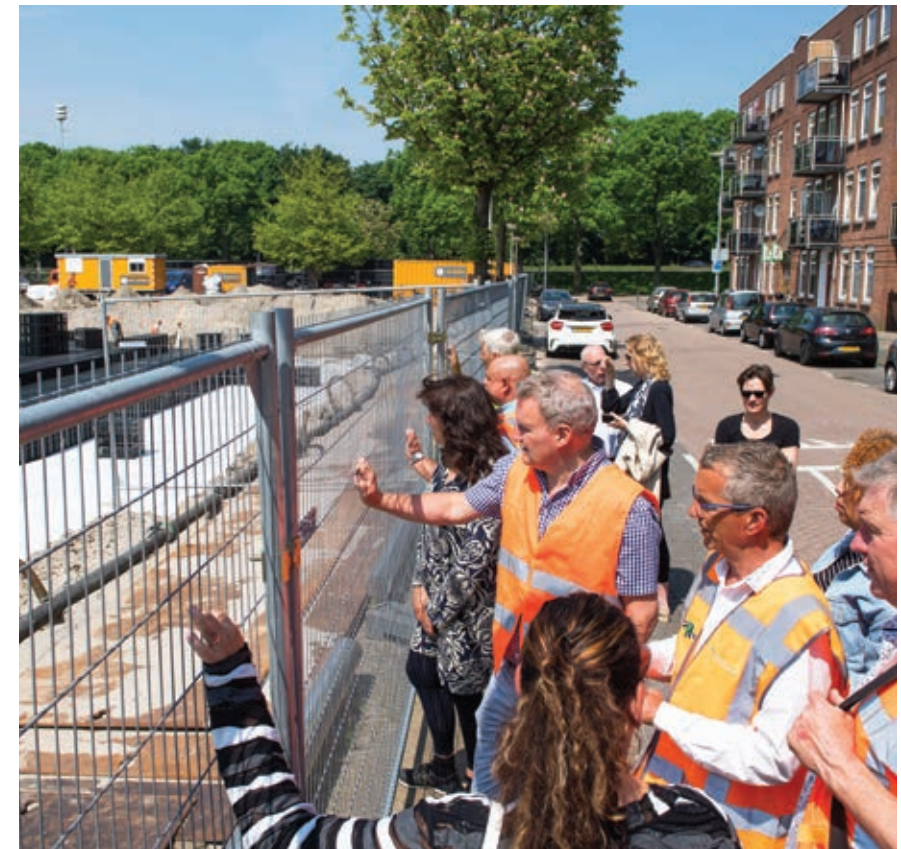
Involving residents and businesses in the redesign of neighbourhoods raises levels of awareness on the impacts of climate change, thereby improving community resilience.
