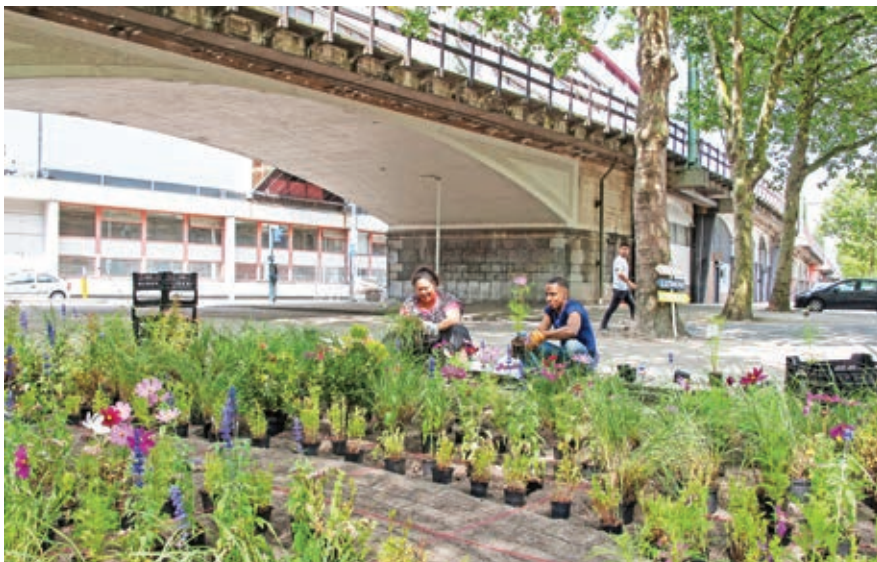
Paved surfaces in ZOHO were converted to raingardens to reduce heat island effect and address excessive rain events.
