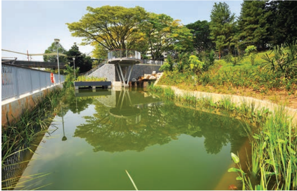
Sedimentation basin at Sungai Ulu Pandan.
