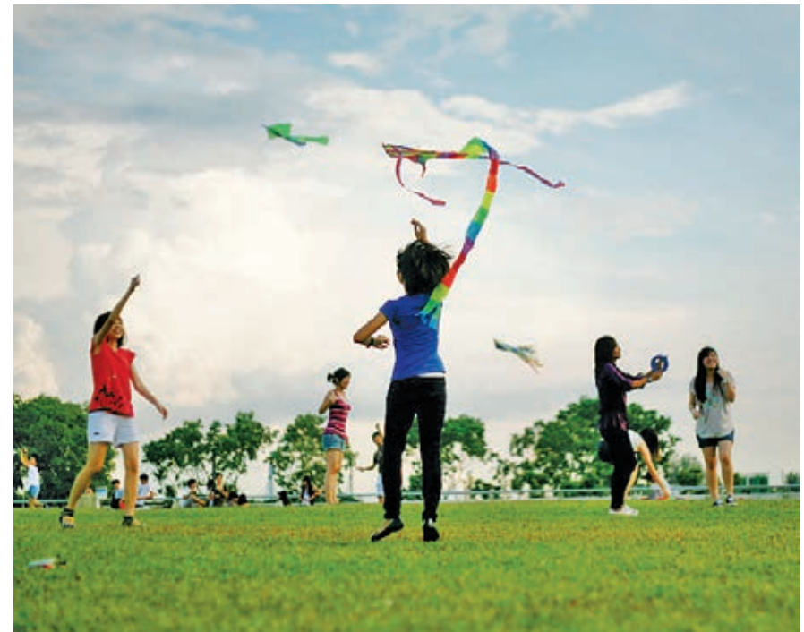
Beyond a pumping station, Marina Barrage was built to double as a recreational space; the rooftop is now a popular kite flying spot in downtown Singapore.
