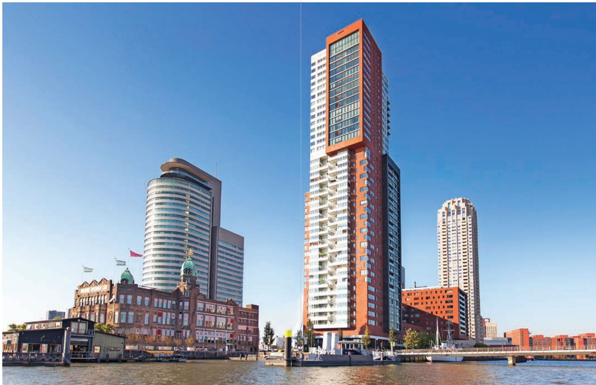
Approximately 85% of Rotterdam is less than 5 m above mean sea level, putting neighbourhoods under flood risk.
