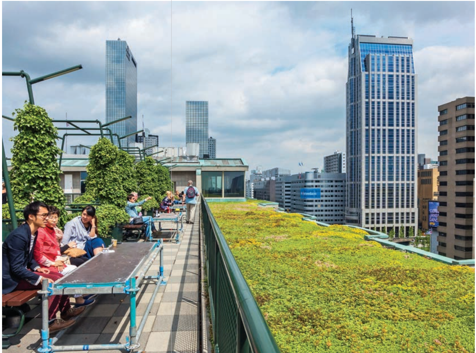
A green roof that retains water next to the Rotterdam central railway station.
