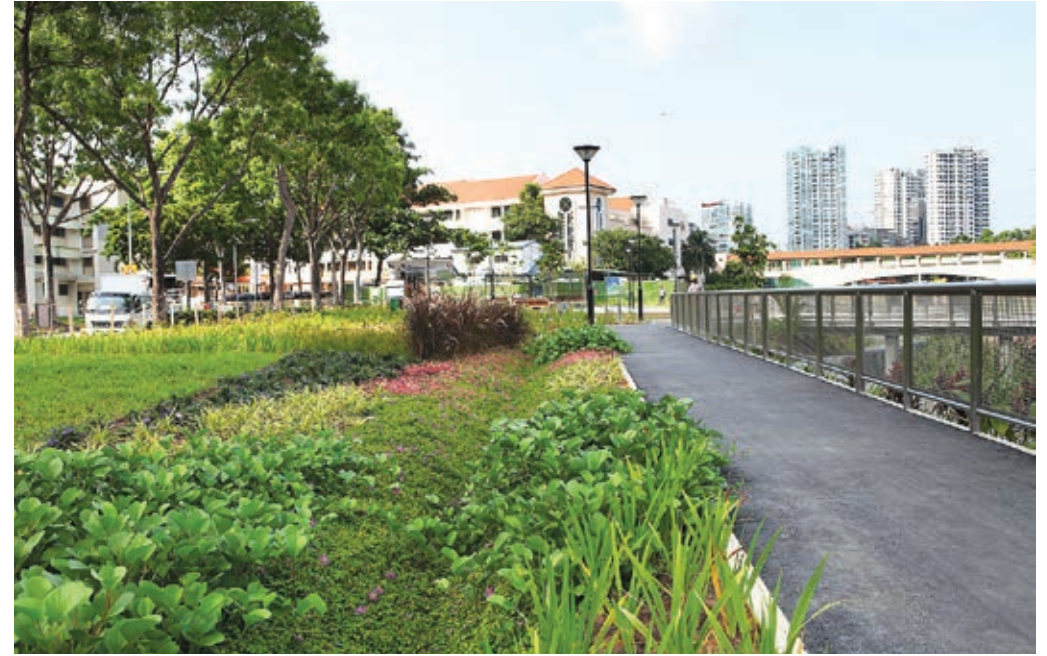
Vegetated swale and rain garden at Kallang River, Potong Pasir.
