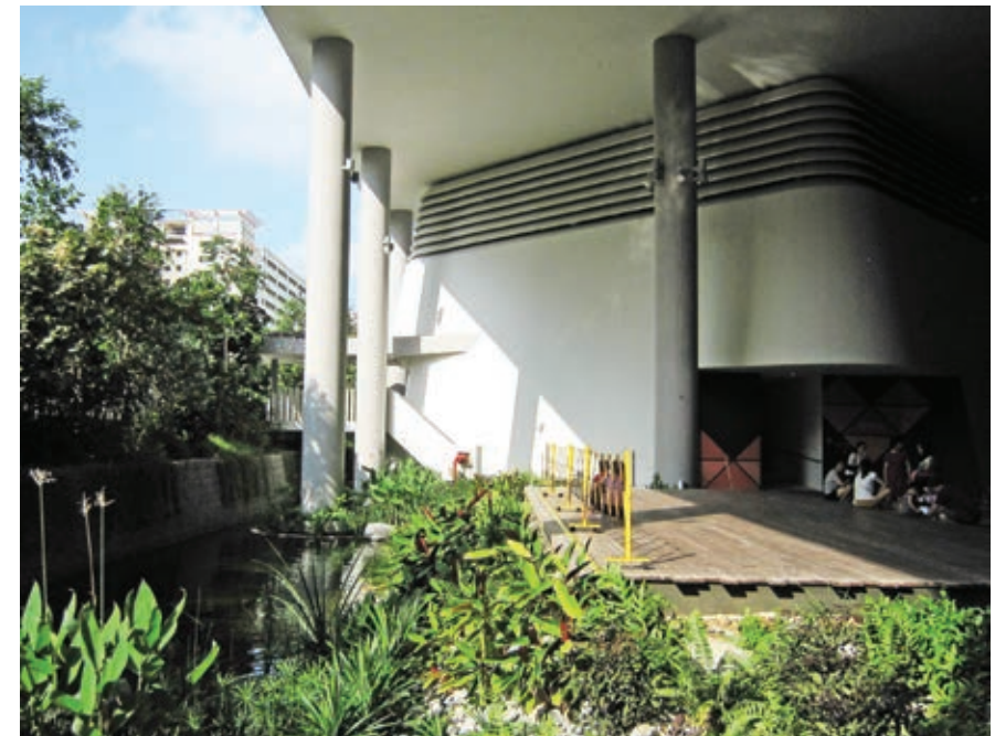
Developments, such as this in Kampung Admiralty, had water harvesting tanks built in from the start to promote water sustainability.
