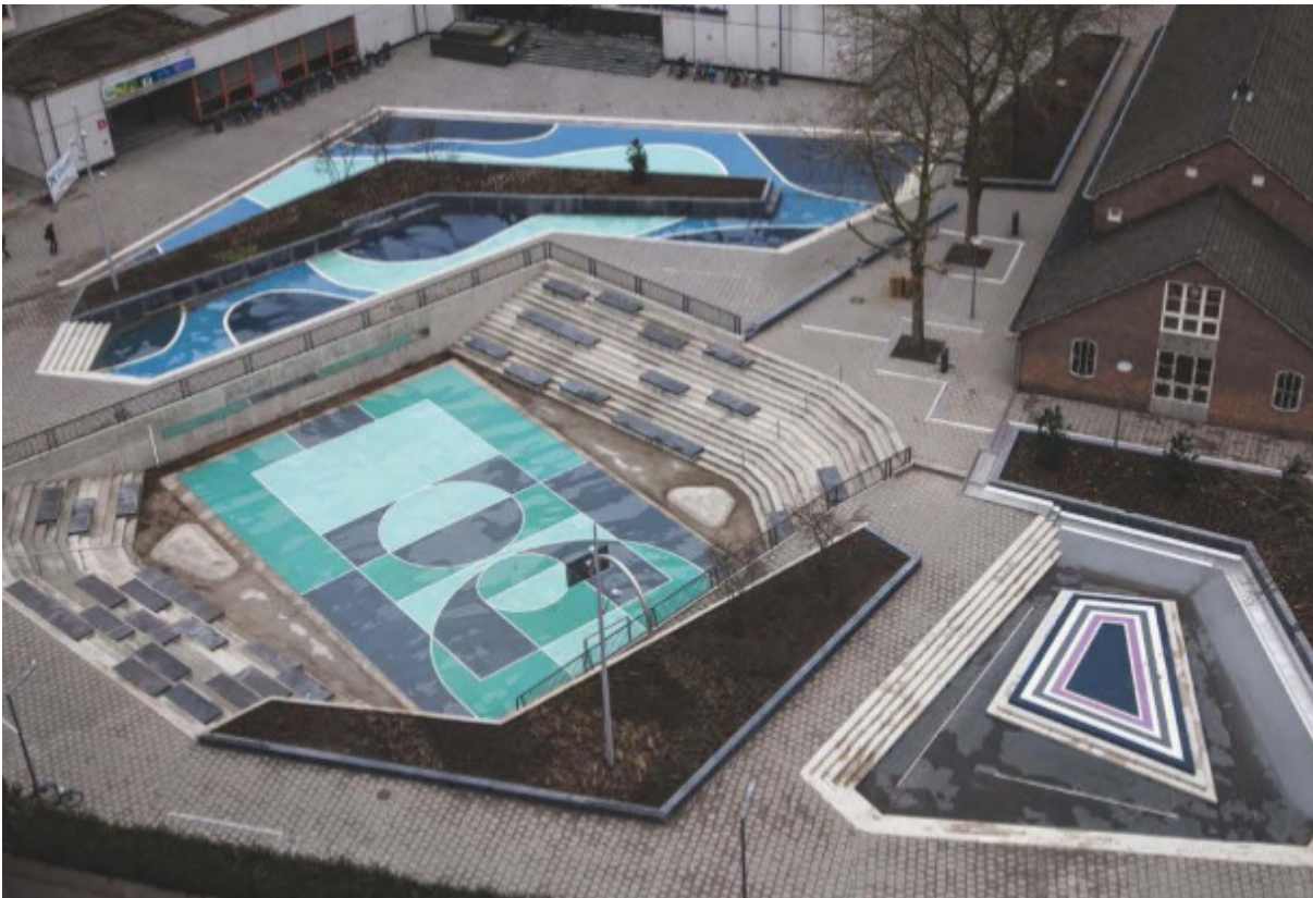
The water plaza in Rotterdam allows for natural flooding during rains and activities when it is dry
