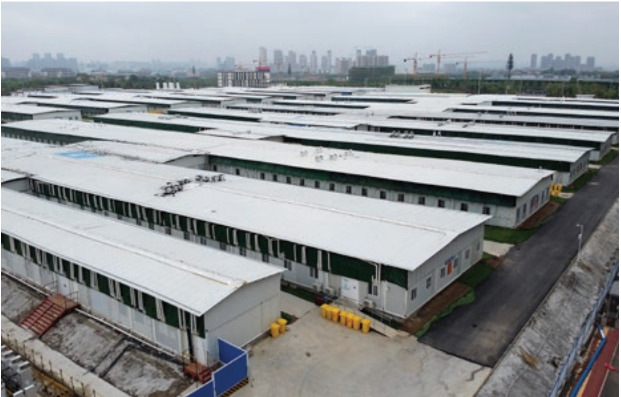
Aerial view of the Leishenshan Hospital in April 2020. Image: Noel Celis / AFP via Getty Images
