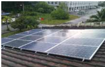
Rooftop installation at Telok Intan, Malaysia
