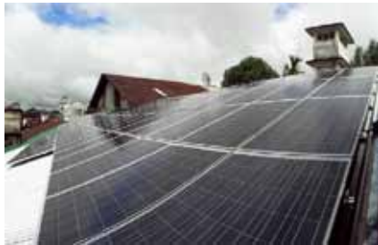
Rooftop installation at Dawei, Myanmar
