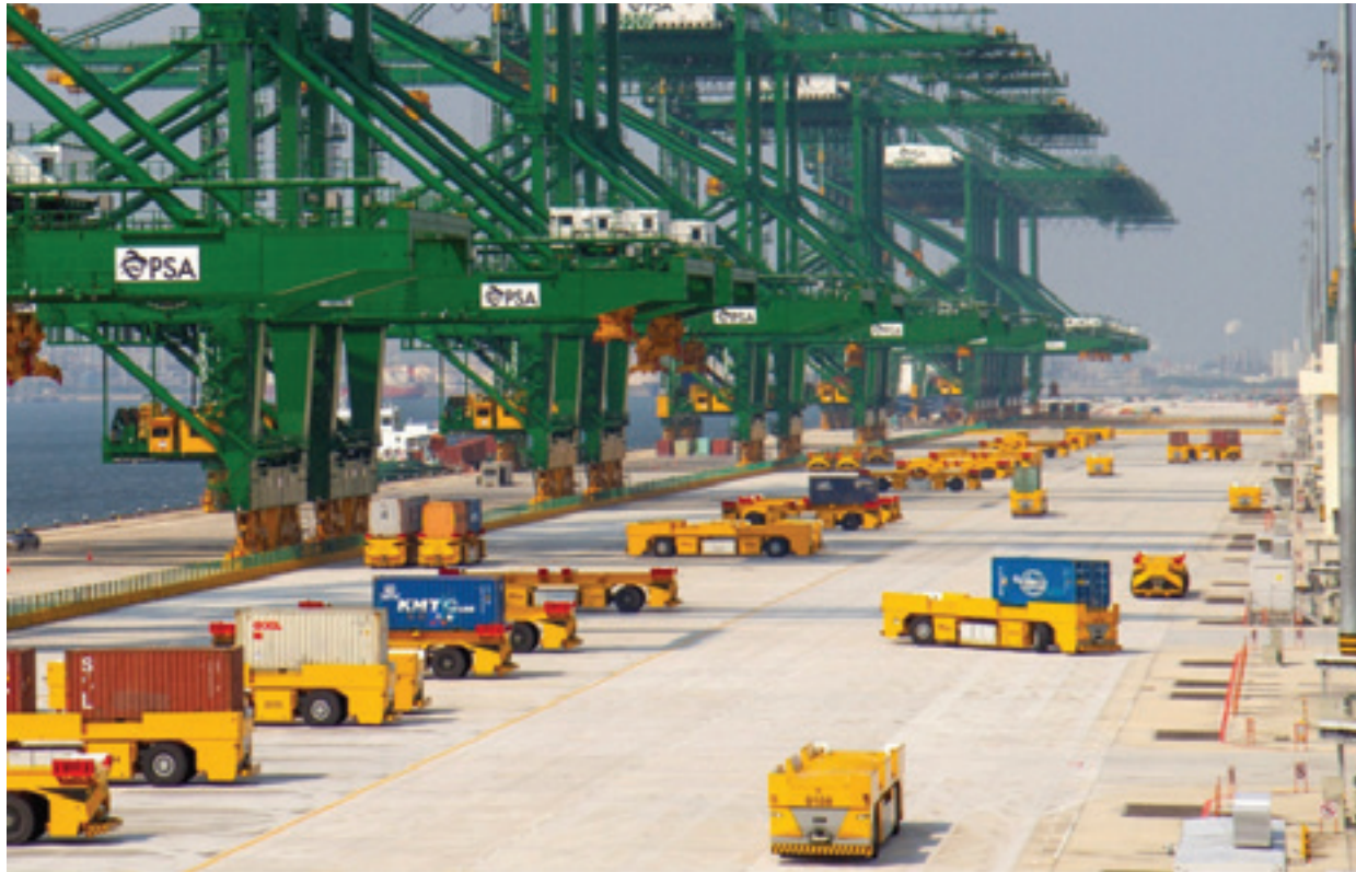
Tuas port will feature smart technologies such as automated yard cranes, drones, and electric and driverless automated guided vehicles. Image: PSA Singapore
