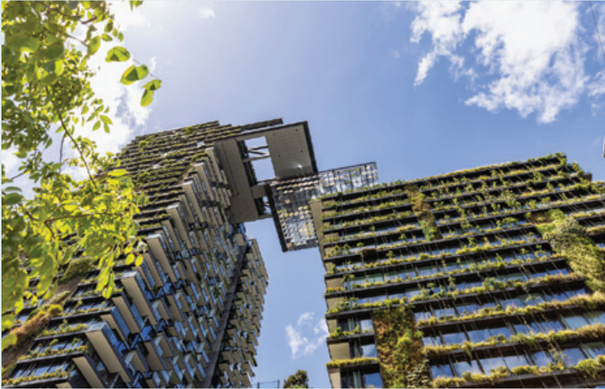
Low angle view of apartment buildings with vertical gardens and heliostat with motorised mirrors, Central Park residential building on Broadway, Sydney, Australia. Image: mamember / iStock
