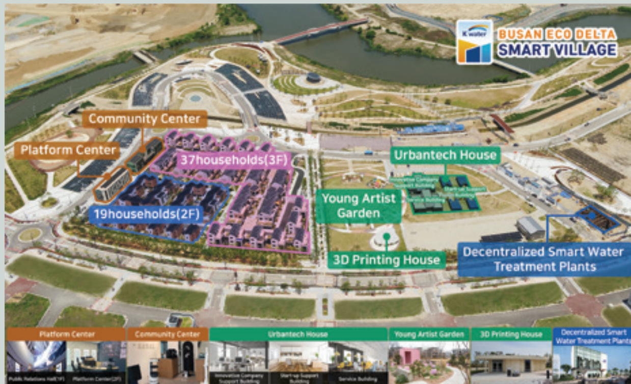
First residential complex of the Smart City—drone view of the Smart Village. Image: Korea Water Resources Corporation
