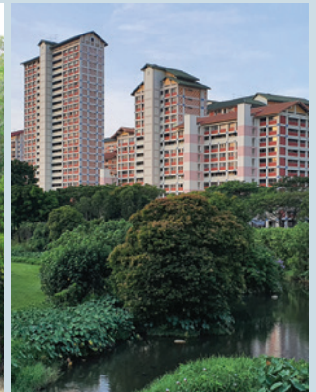
The naturalised waterway at Bishan-Ang Mo Kio Park serves as a nature-based solution to build resilience against inland flooding, while providing additional benefits as a biodiversity habitat and recreation area. Image: National Parks Board
