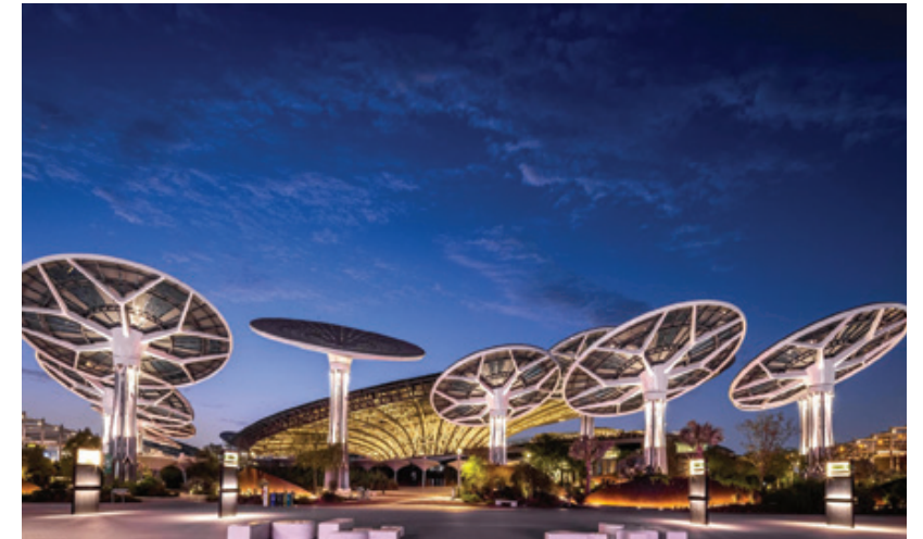
Expo City Dubai aims to be a model for a sustainable and smart built environment through passive design strategies and technology-based solutions. Image: Expo City Dubai
