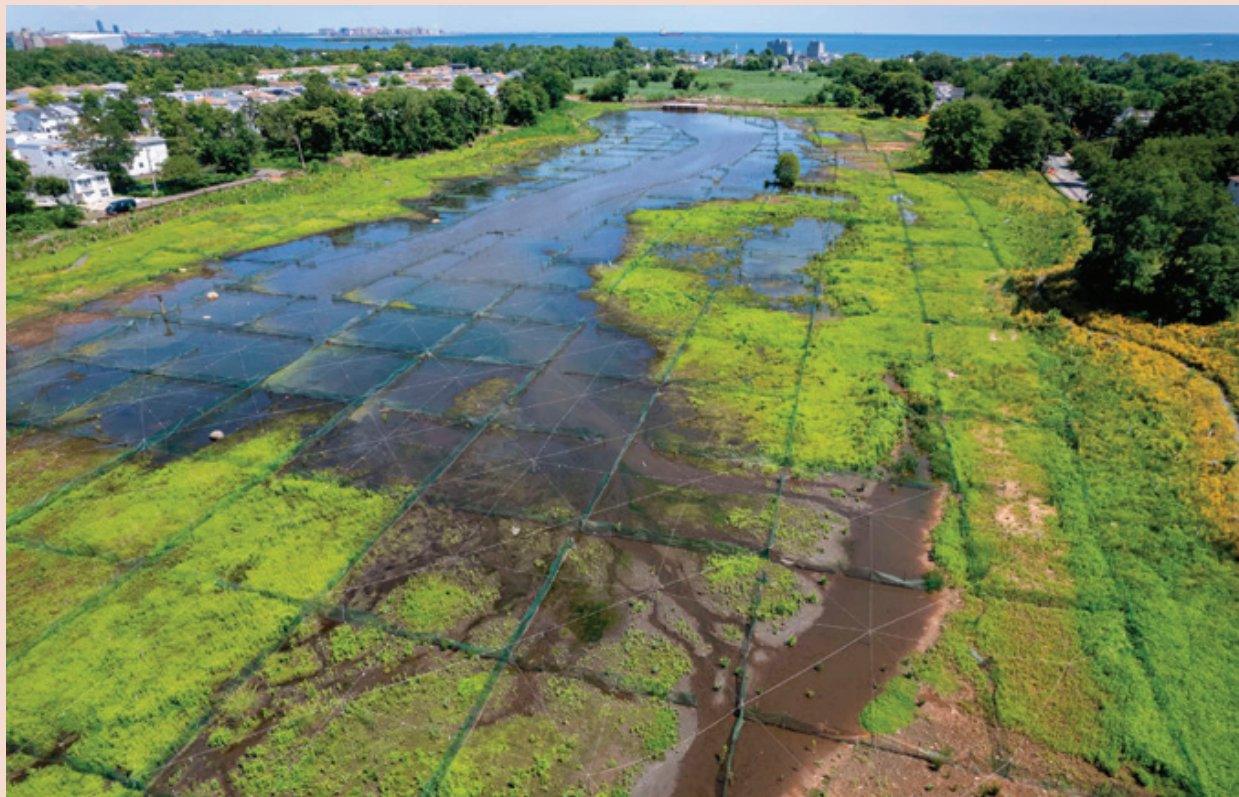
New Creek Bluebelt Olympia Boulevard portion, taken in July 2024. Image: NYC DEP
