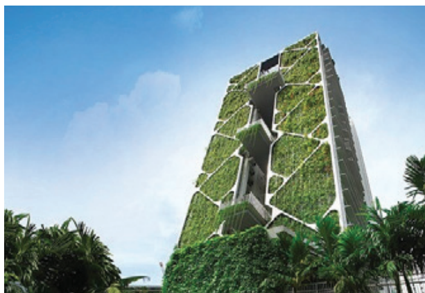
CDL Tree House Condominium, completed in 2014, embodies extensive adoption of nature-based solutions. Image: City Developments Limited
