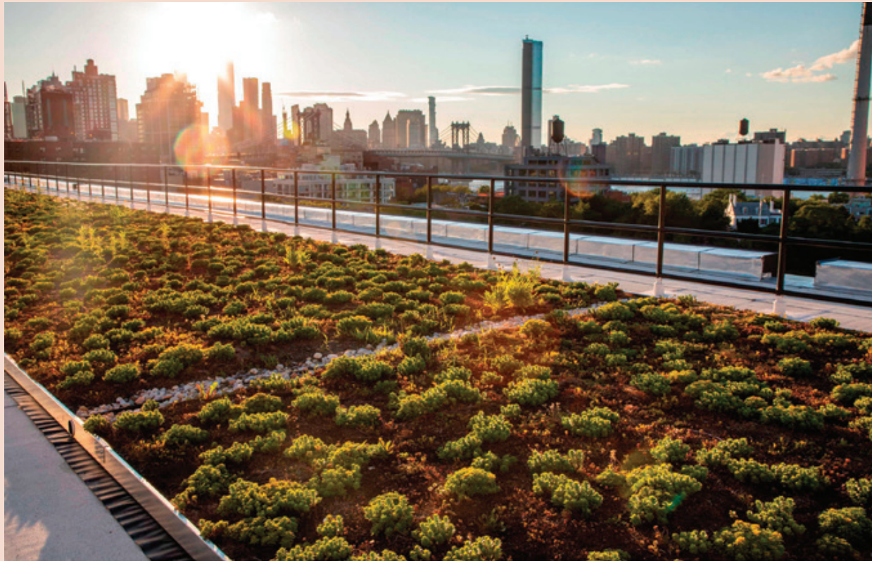
Green roof on Steiner Studios, Brooklyn Navy Yard. Green roofs help infiltrate rainwater, reducing peak flows from the sewer system. Image: NYC DEP
