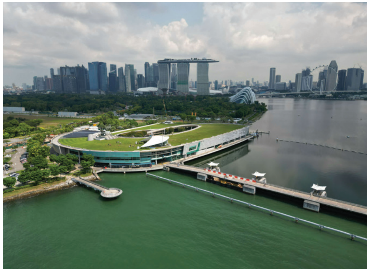
The Marina Barrage serves as a source of water for Singapore, provides flood control for low-lying urban areas, and is a venue for lifestyle attractions. Image: Bob Tan / Wikimedia Commons
