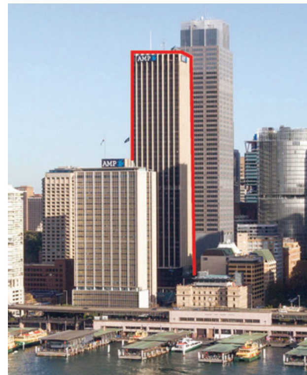
Old and rejuvenated AMP Building. Image: City of Sydney
