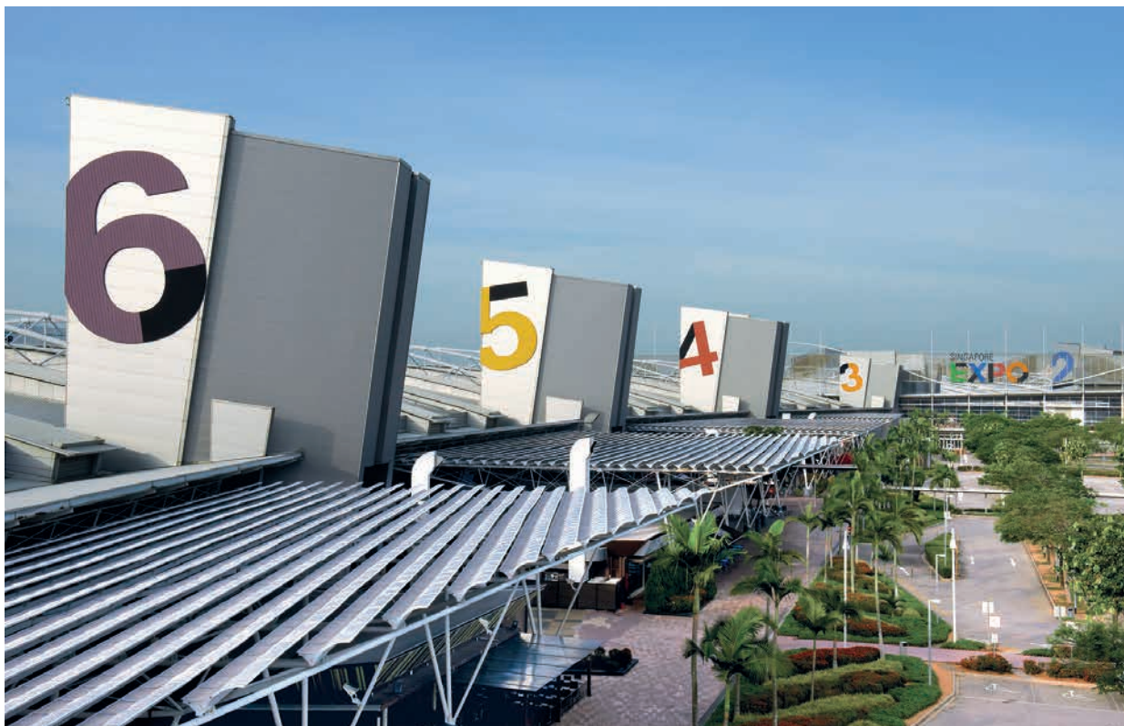
The Singapore Expo Convention Centre's ten exhibition halls were temporarily converted into a care facility for COVID-19 patients in April 2020. Image: SingEx-Sphere Holdings Pte Ltd
