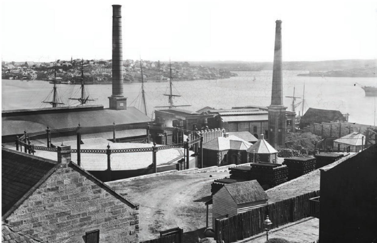
Millers Point Gasworks brought the first coal gas street lights to Sydney but left East Darling Harbour contaminated with large deposits of coal tar. Image: Mitchell Library, State Library of New South Wales
