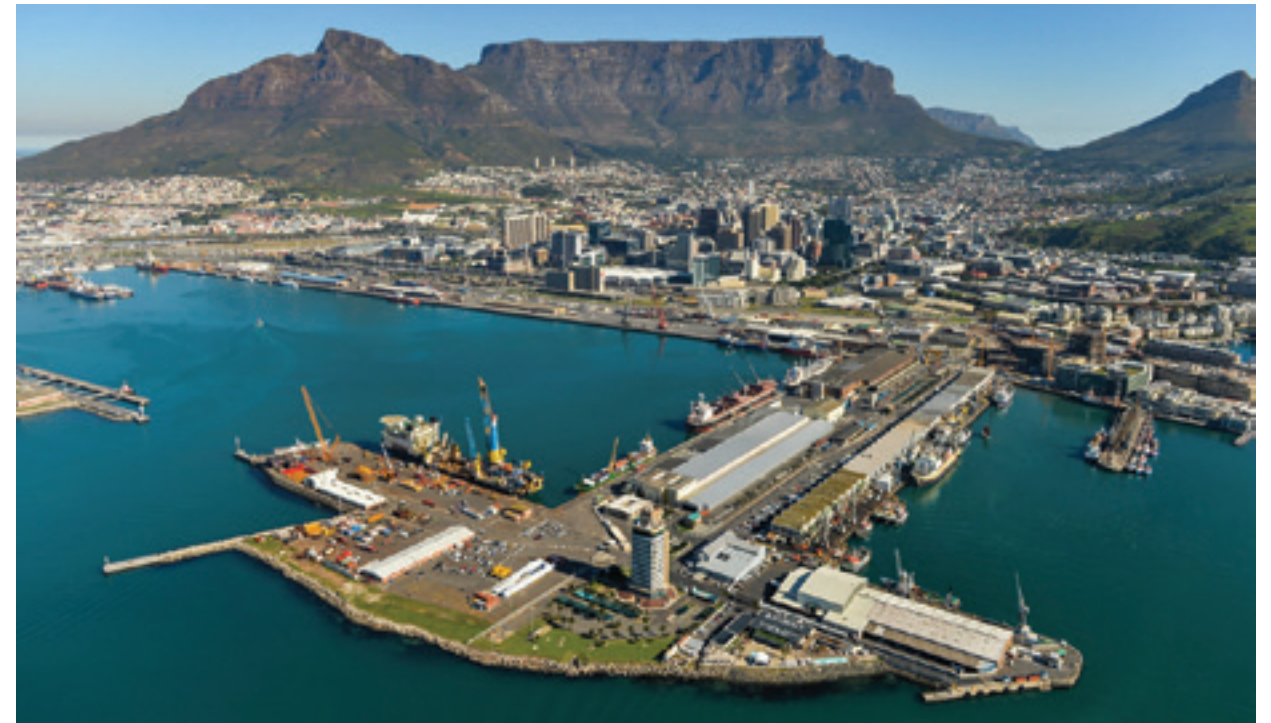
Aerial view of Port of Cape Town. Image: City of Cape Town
