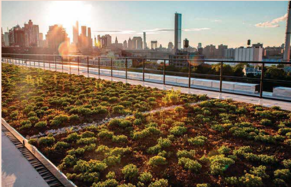
Green roof on Steiner Studios, Brooklyn Navy Yard. Green roofs help infiltrate rainwater, reducing peak flows from the sewer system. Image: NYC DEP
