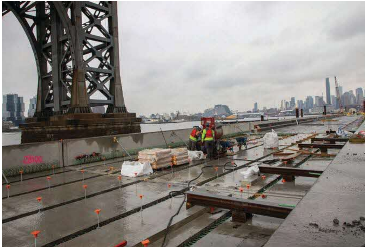
Construction of elevated East River Park as part of the ESCR project along the East River in lower Manhattan. Image: NYC Department of Environmental Protection
