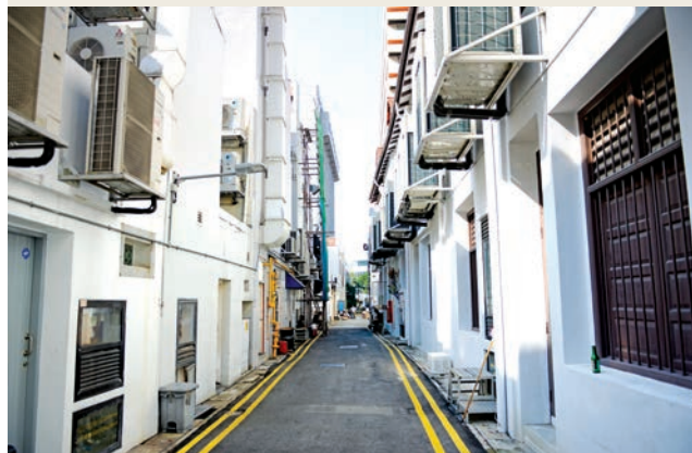
Service back lane created between two rows of shophouses at Tanjong Pagar. Courtesy of Cheong Kay Teck.
