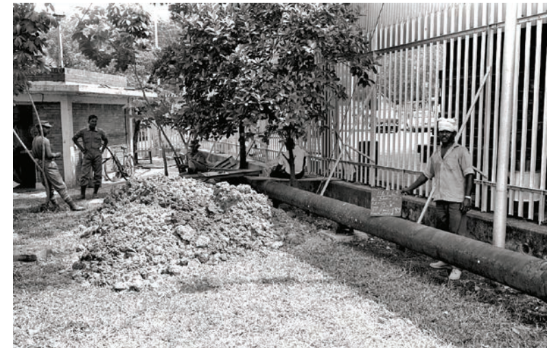
Electricians laying the underground cables.
