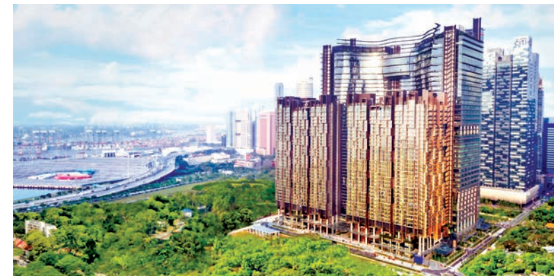
Marina One—A Green Mark Platinum non-residential building. Courtesy of M+S Pte. Ltd.
