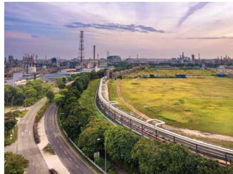
11. Chemical and utility pipelines as seen on Jurong Island today.
