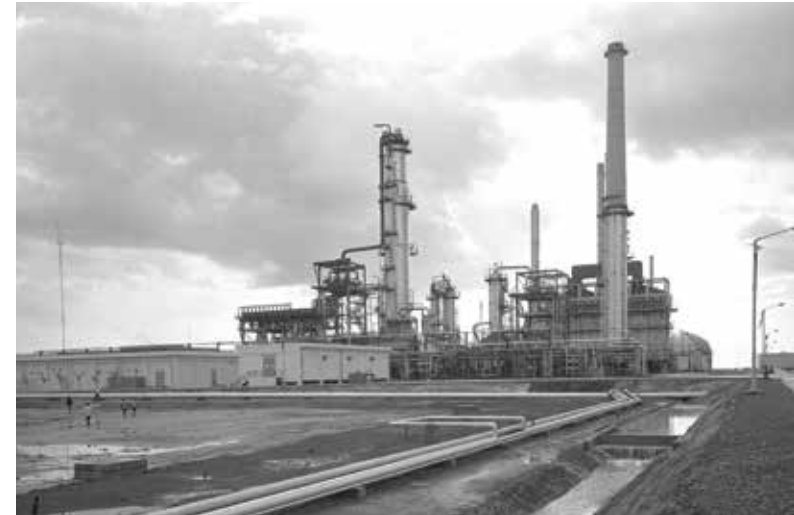
5. Esso Refinery at Pulau Ayer Chawan, off Jurong, 1971.
