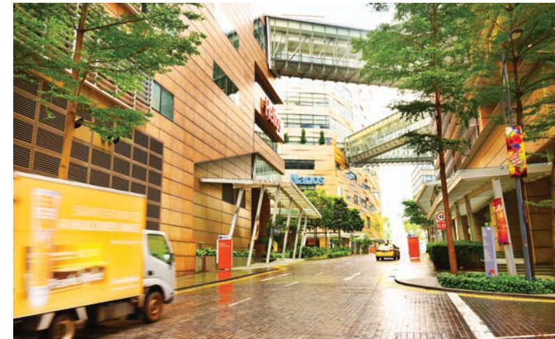
Narrowed road widths and honed granite cobblestones at Biopolis as traffic calming measures.
