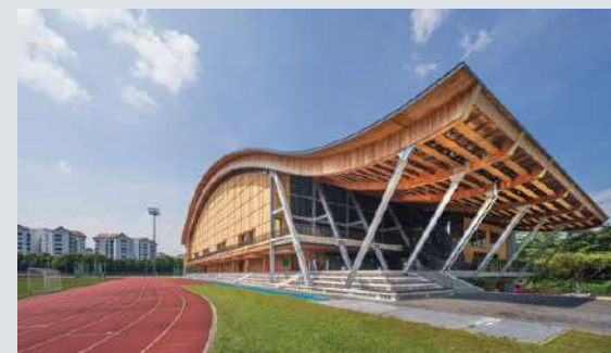
29. The Wave at NTU is one of the first large-scale buildings in Southeast Asia built using MET; the large roof did not require any internal columns, leaving a cavernous 3-storey space.
