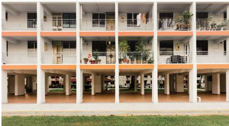
19. The HDB flats were built with windows that orient north-south to promote cross ventilation and have void decks to draw wind onto the ground and improve wind flow. 98
