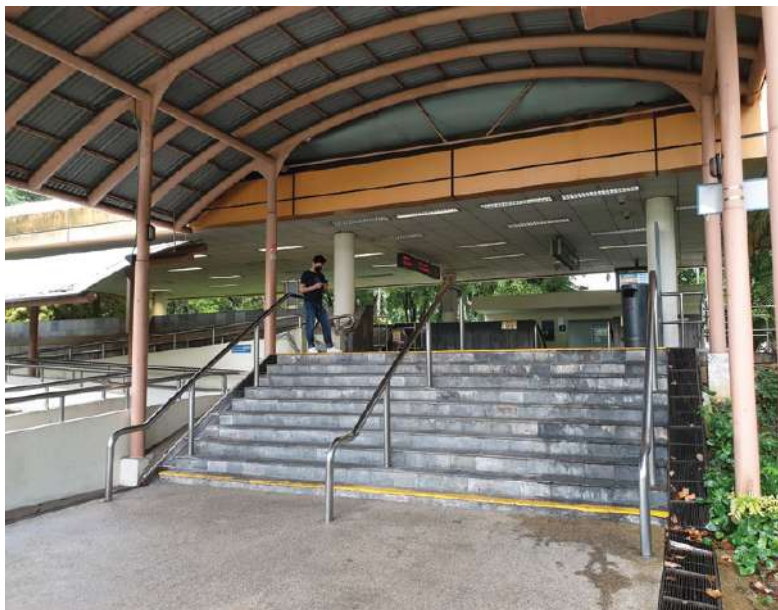
34. Entrances of MRT stations are elevated to reduce flood risk in times of intense rainstorms.
