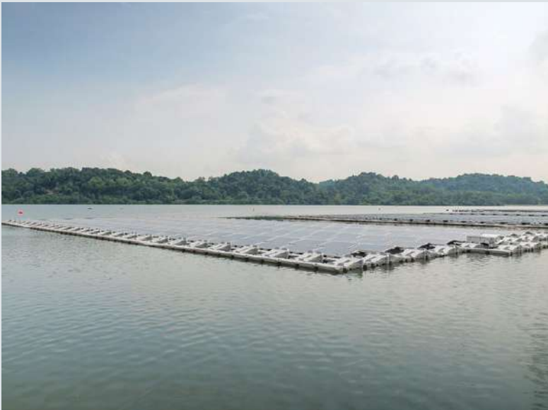
28. In 2016, the PUB and EDB launched a 1 MWp testbed at Tengeh Reservoir to study the feasibility of floating solar PV deployment on reservoirs.
