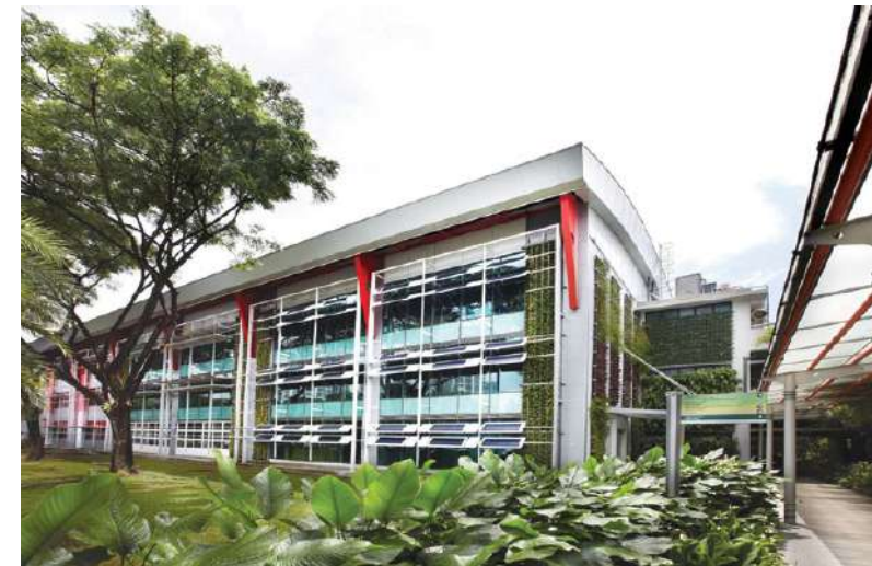
24. The BCA's Zero Energy building is a prototype that is a model for developers and builders to learn from.
